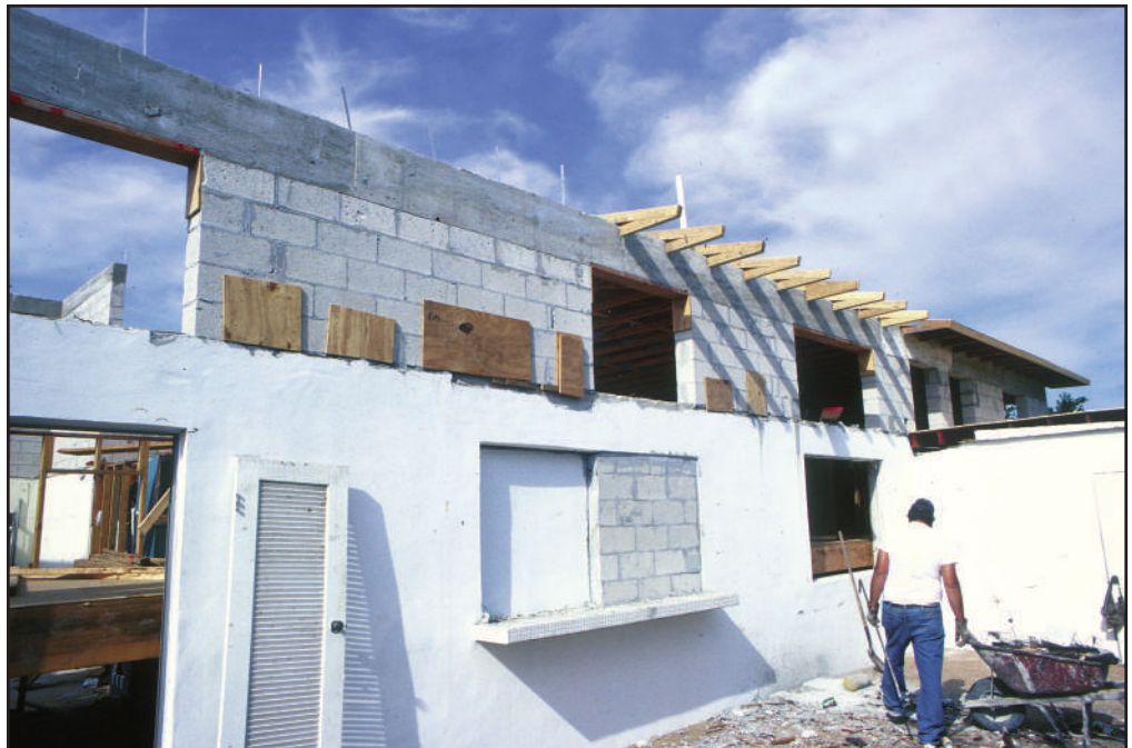
Figure 67 The extended first-story walls.
