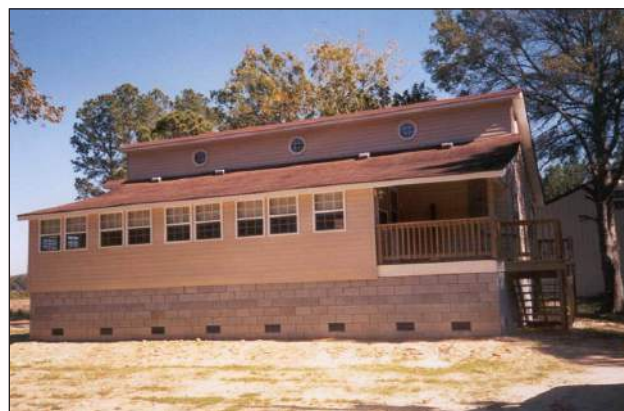
Figure 3-7. Before (left) and after (right) photos of a retrofitted home elevated on extended continuous foundation walls.
