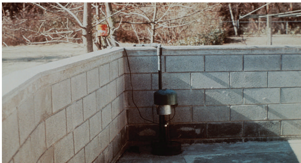
Figure 8-6. Small patio floodwall with sump pump.
