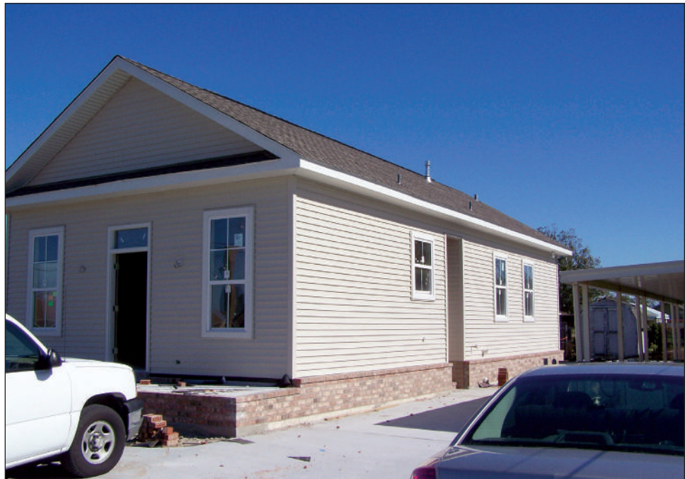
Figure 6-9. Typical mitigation reconstruction project.
