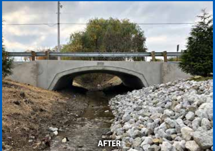
Streambanks reestablished under bridge.
