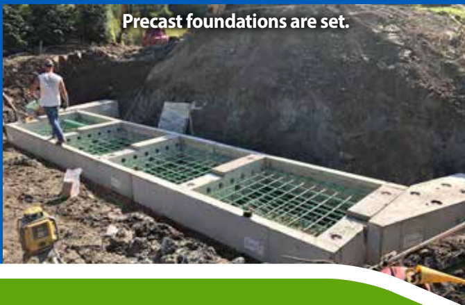
Excavation for the new precast foundations.
