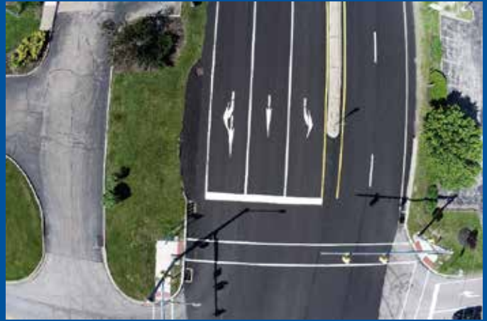
Douglas Parkway Repaving Project
