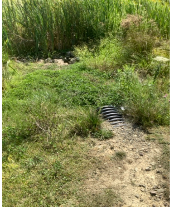
Photo # 14. Pipe inlet to rain garden.
