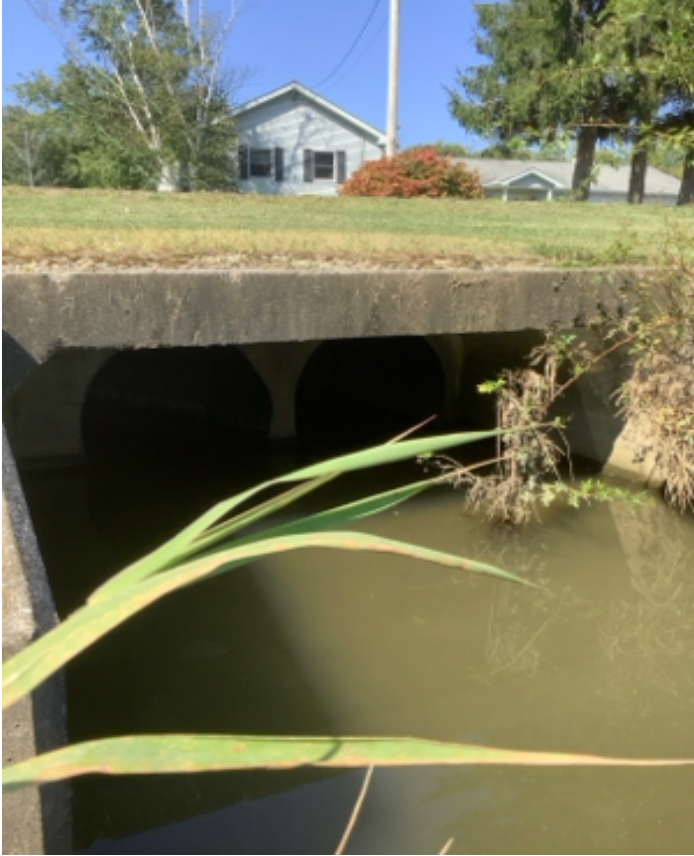
Photo # 11. Discharge pipe outlet into LeBoeuf tributary, across Old French Road. Detention BMP will discharge through left outlet.
