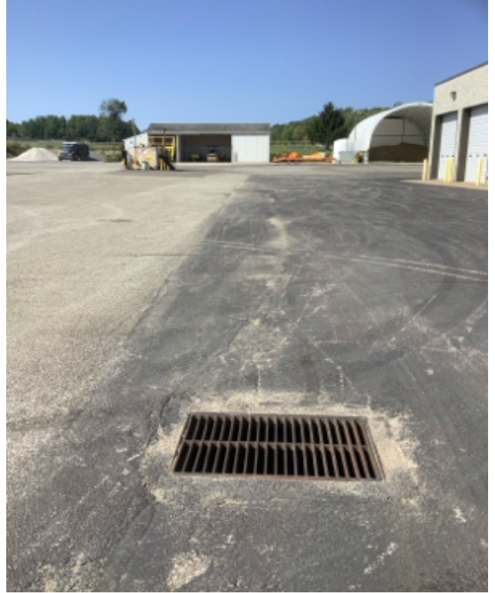
Photo # 8. A series of catch basins lead from the direction of fuel station to underground detention BMP.
